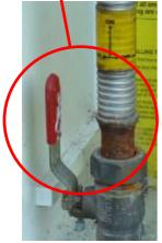
With the door open you will see a gas meter and associated pipework. On one of the pipes will be a handle that can turn 90 degrees. With the handle in line with the pipe the supply is on. Turning the handle so it is at right angles to the pipe will turn the supply OFF.
